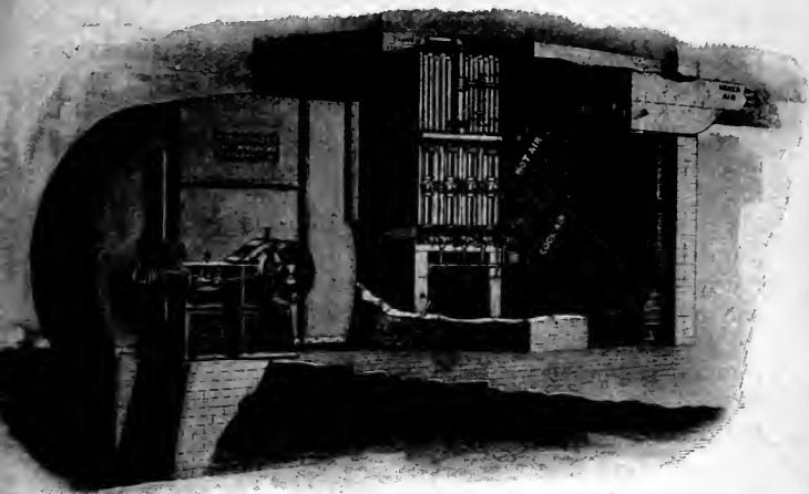
Three-Quarter Housing Fan, Left-Hand Top Horizontal Discharge, Blowing Air Through and Underneath Heater into Brick Plenum Chamber
